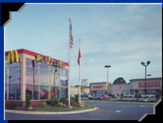
Oakwood Square Greensboro, NC
